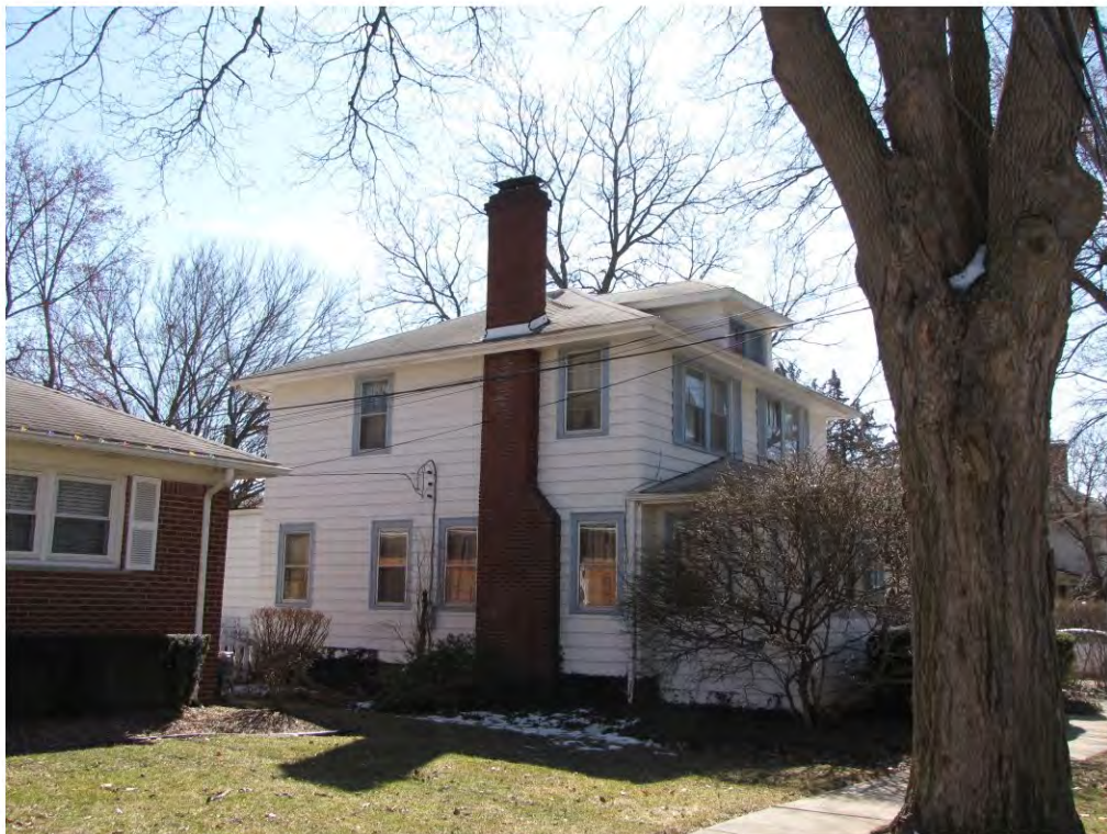
West 114_Looking Southeast
