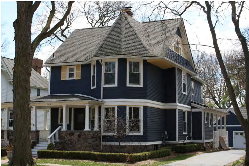
Dunlap West 543_Looking Southeast
