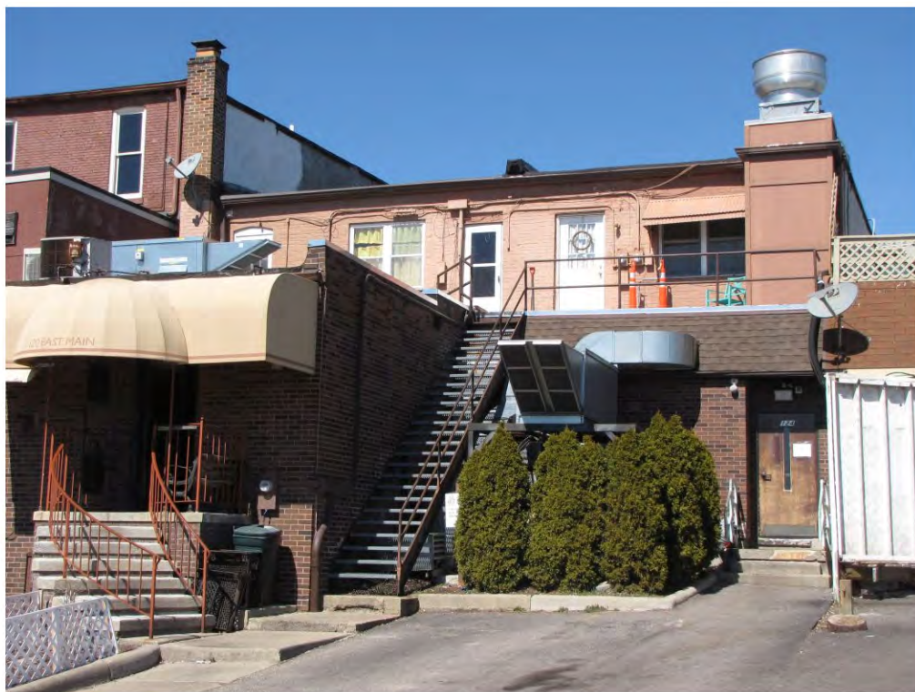
Main East 120-124_Looking Northwest
