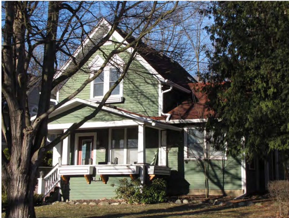
Rogers North 359_Looking Southwest
