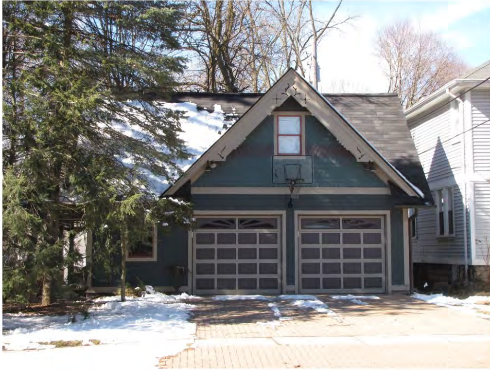
Dunlap West 504, Garage_Looking West
