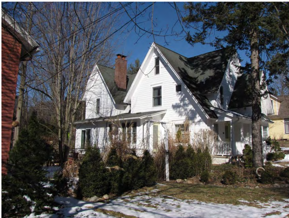
Rogers North 207_Looking Northwest
