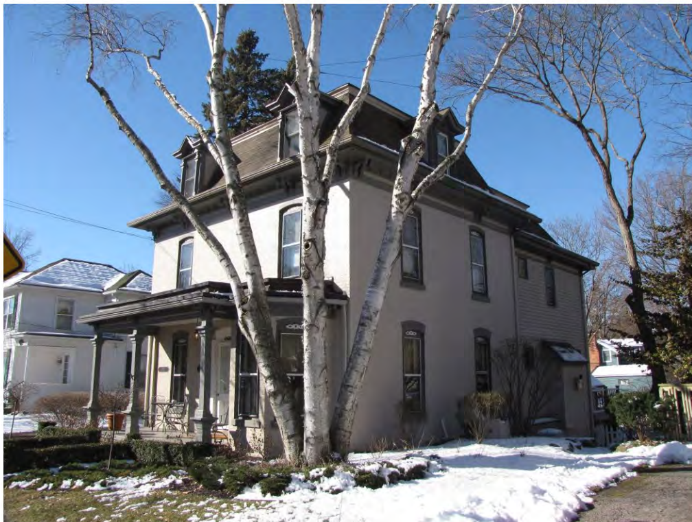
Rogers North 109_Looking Southwest
