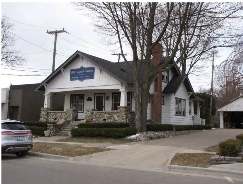
Wing North 111_Looking Southwest
