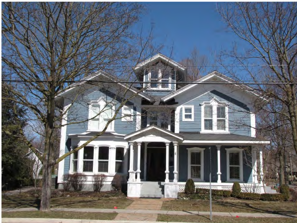
Main West 404_Looking North
