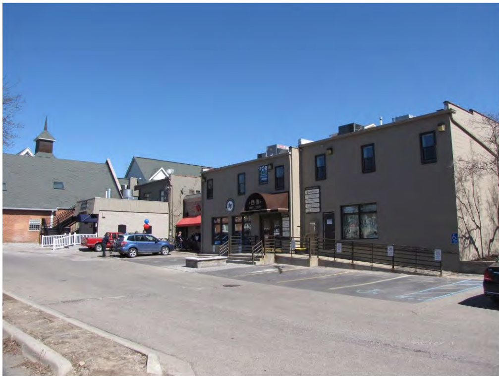
Center North 109-115_Looking Northeast
