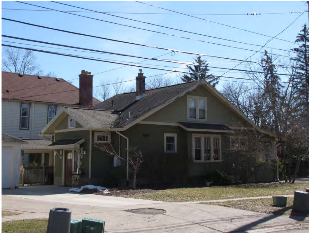
Dunlap West 314_Looking Southeast
