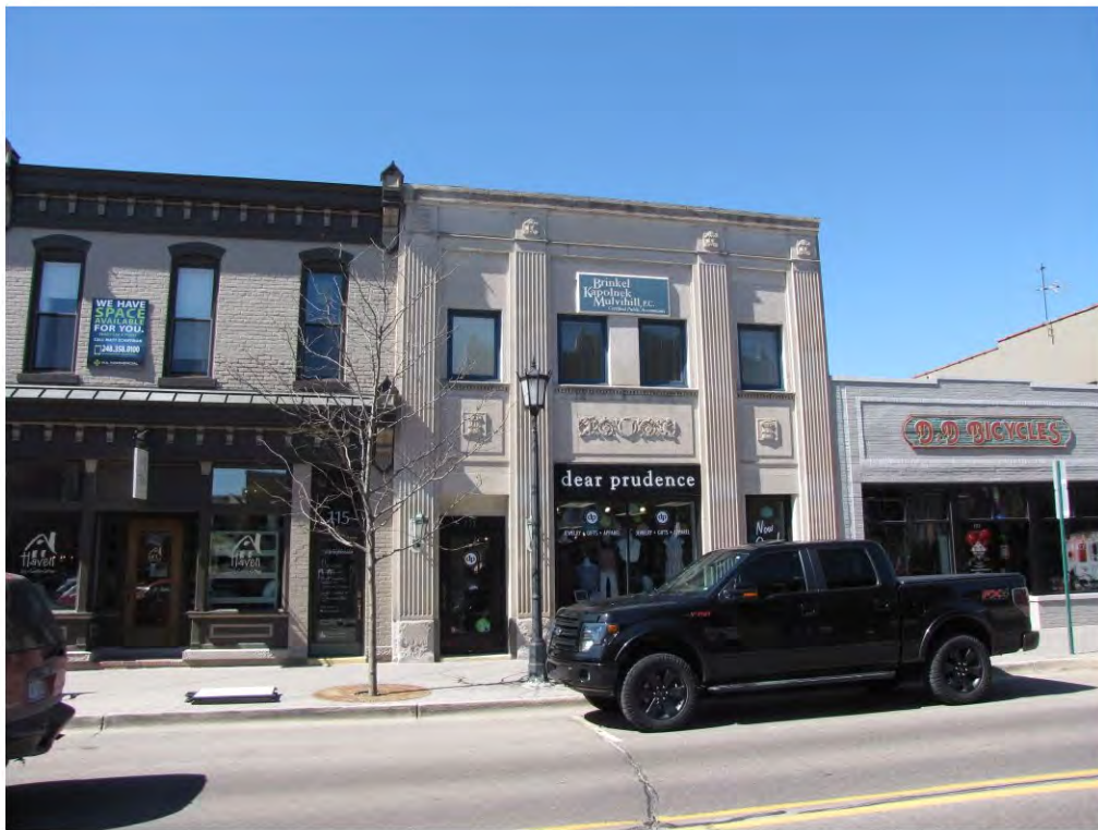
Center North 119_Looking Northeast
