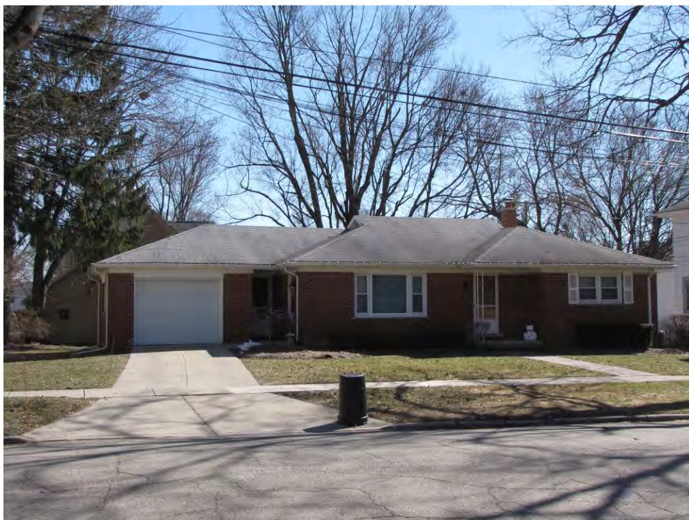
West 120_Looking Southeast
