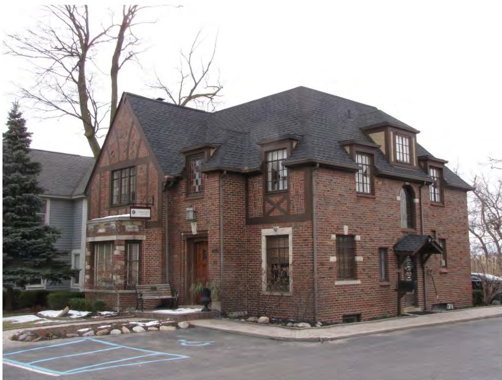
Main East 324_Looking Southeast
